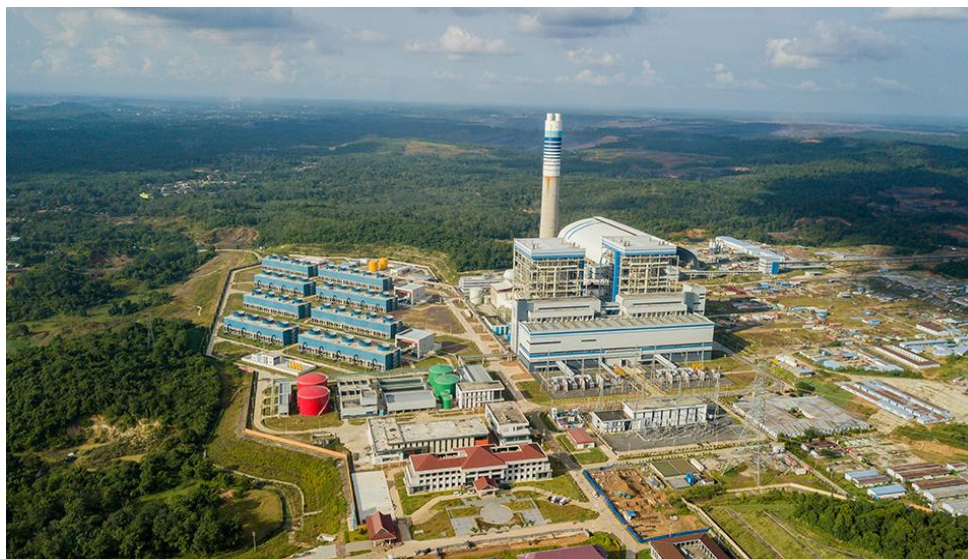
Figure 54. Sumsel-8 steam power plant
