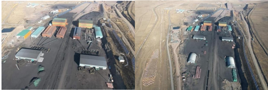
Figure 5 Factory of improved briquette fuel
